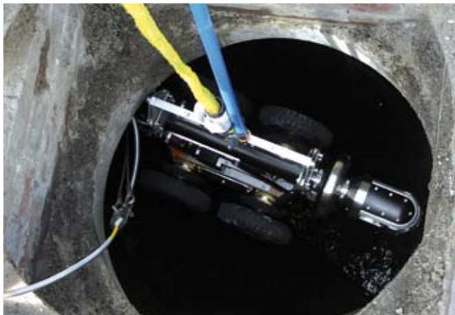
Figure 5.7: Lowering the crawler into a manhole
