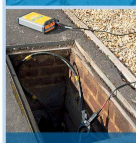
Signal clamping (Optional) Applies a transmitter signal safely to a pipe or live cable up to 125mm/5" diameter without interrupting the supply.
