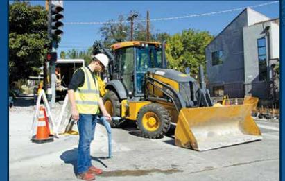
**Interference** is an electrical disturbance that can affect the accuracy of the locator, typically caused by substations and buried or overhead high voltage cables
